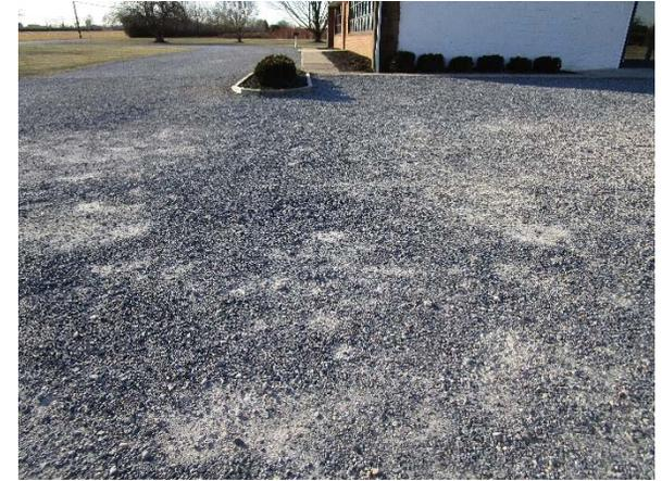
Parking spaces east of the church can be replaced with pervious pavement to capture and infiltrate stormwater runoff from the lot and rooftop runoff from the church. A preliminary soil assessment suggests that more soil testing would be required before determining the soil's suitability for green infrastructure.
